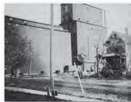
14 2845 10TH AVENUE SOUTH: ELEVATOR X
